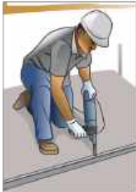
Step 01 Framing (Tracks)
