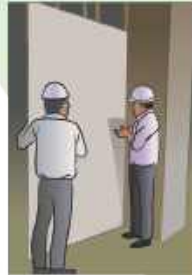
Step 03 First side board fixing
